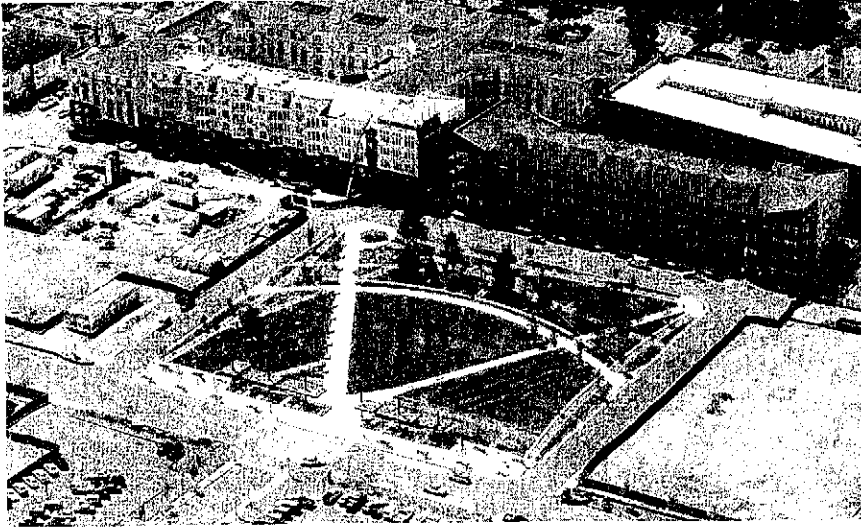
Figure 8-15 The 2.2-acre green at Belmar, occupying a full block and located on axis with Teller, the main north-south street, is a quiet place.
